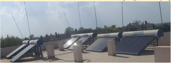
A typical solar water heating system can save up to 1500 units of electricity every year, for every 100 liters per day of solar water heating capacity.
